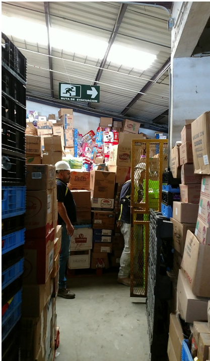
Means of egress not protected in any way
