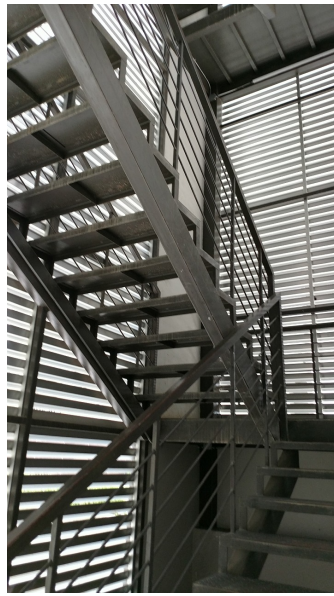
Open main staircase
